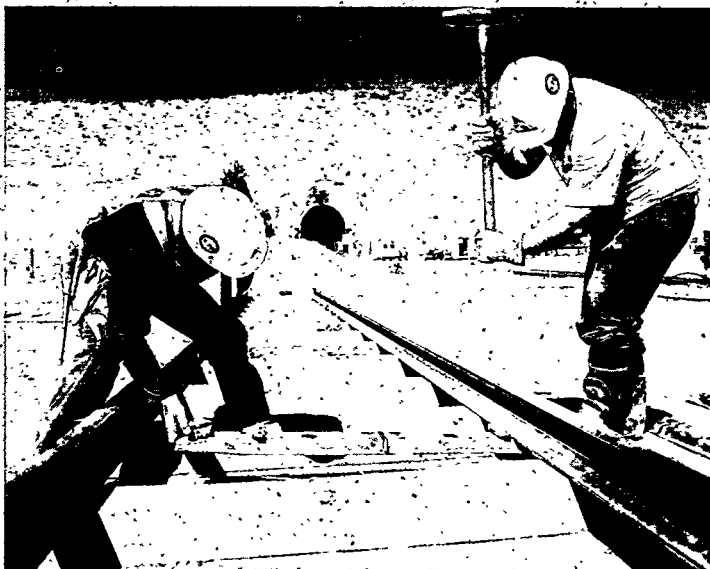
Layin' 'em in and tyin' 'em down... Workers run a track for muck cars into the TBM starter tunnel. Current TBM technology is a combination of the latest developments and standards such as railroad tracks, which are used when appropriate.
