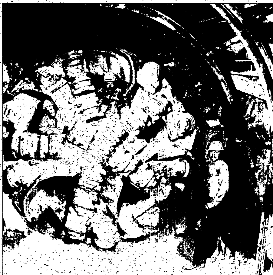
A modern tunnel boring machine, or "mole," breaks through the opening of the Vatt Tunnel in Utah in 1981. (Photo: U.S. Department of the Interior, courtesy of Franklin Watts Photo Archives).
