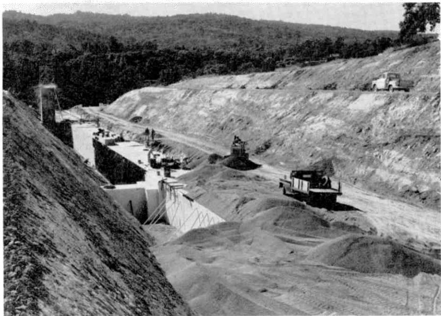
FIG. 30--The first few sections of Accelerator Housing with the pea-gravel back-fill covering the protective Celotex sheets.
