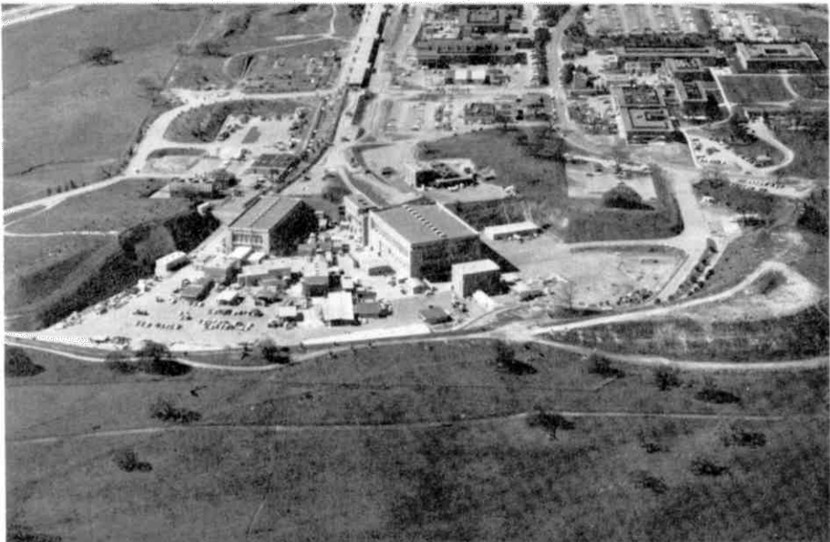
FIG. 53--The research end of the accelerator. The fork-shaped beam switchyard, under 40 feet of earth shielding, directs the accelerator beam to the desired experimental area in the two end station target buildings.
