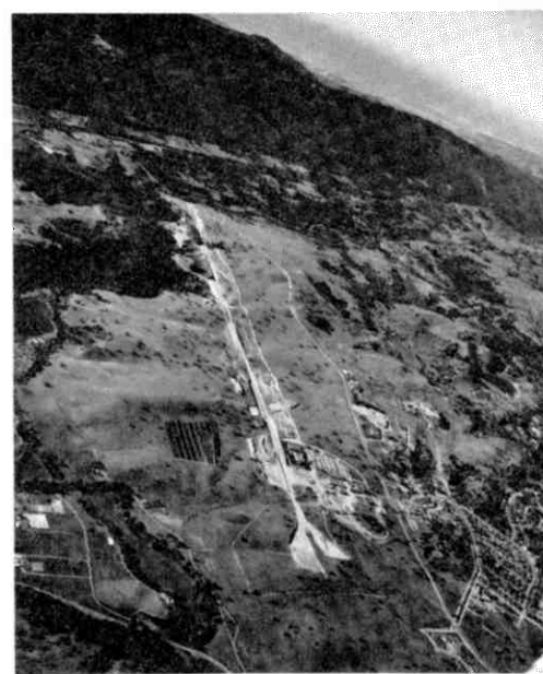
FIG. 27--The two-mile-long cut-and-fill in mid-1964, looking west toward the Pacific Ocean from the initial excavations for the two target buildings.
