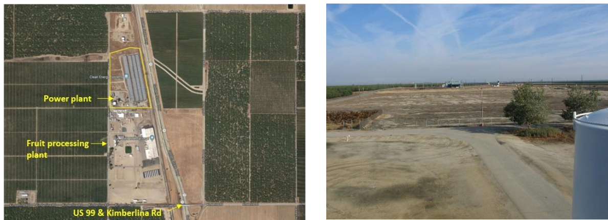
Figure 6-1 Aerial View of the Kimberlina Site (Left) and Area Available for Well Drilling at CES KPP (Right)
