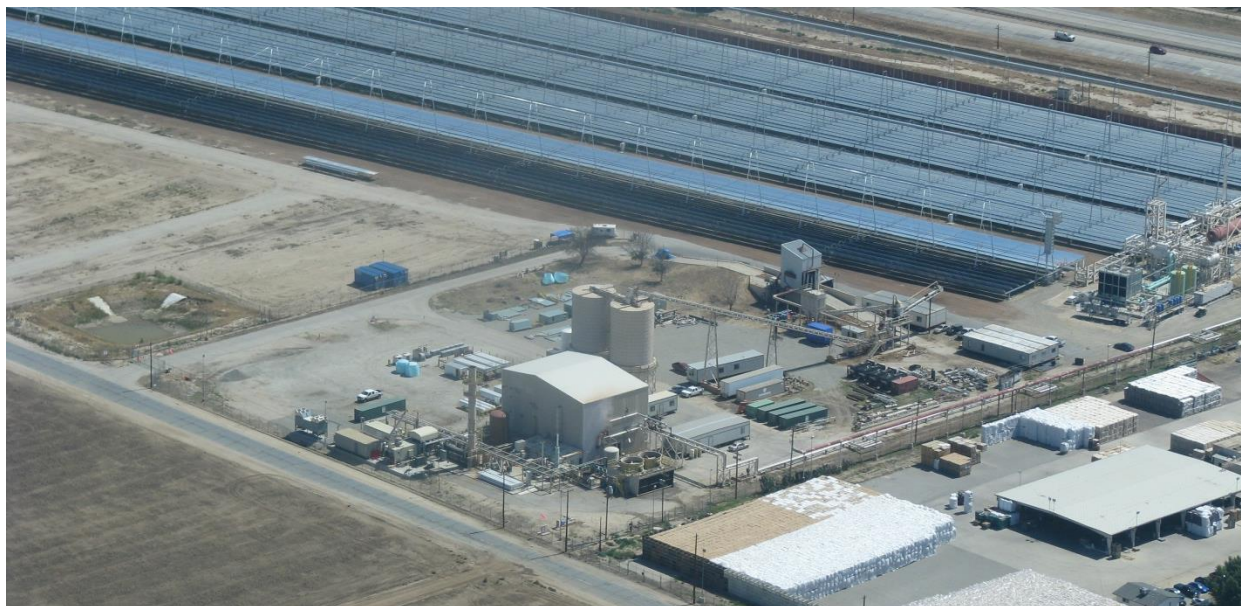
Figure 7-3: Aerial Photograph of the Kimberlina Power Plant
