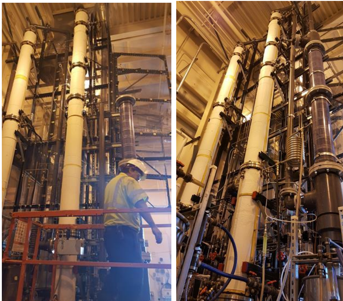
Figure 85. Photographs of the absorber system taken during the water-wash installation (left) and the completed system (right).
