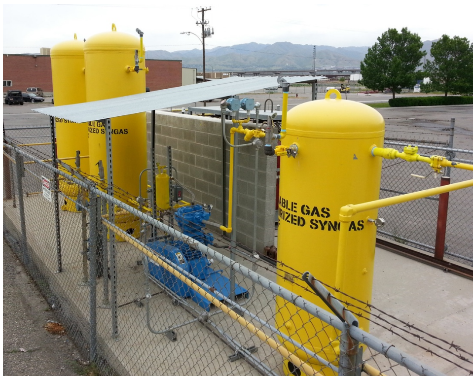
Figure 5. Ceramatec syngas compression system.
