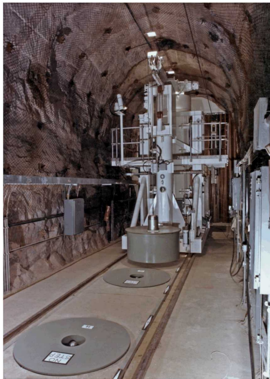
Figure 1. Waste disposal demonstration in granite at the Nevada Test Site (Patrick 1986).
