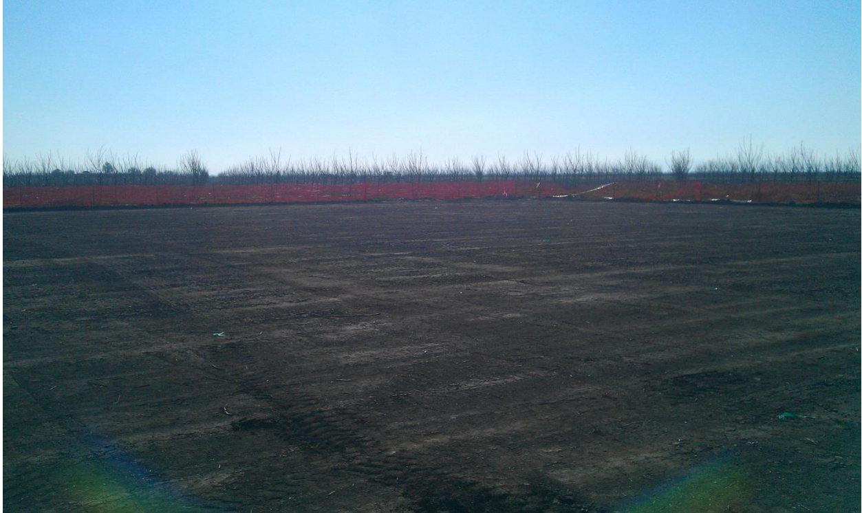
Figure 5-2. Placement of Subgrade, Geotech Fabric, and Initial Compaction
