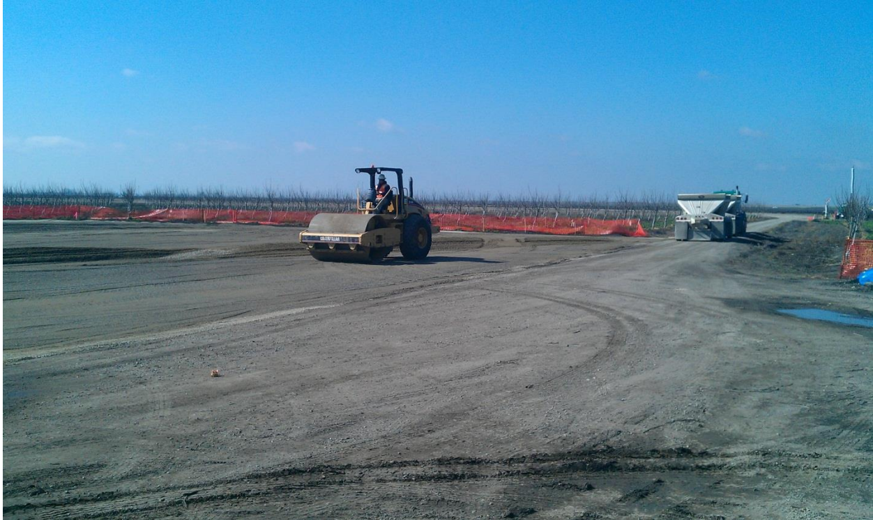
Figure 5-3. Aggregate Placed for Well Pad; Compaction Ongoing
