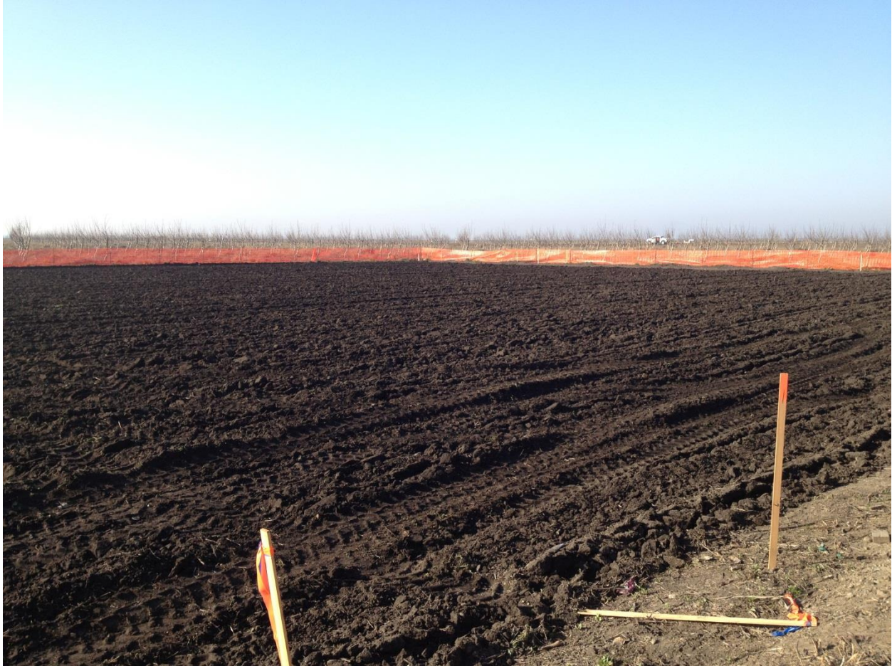
Figure 5-1. Clearing and Grubbing (Removal of Organic Matter) of King Island Site
