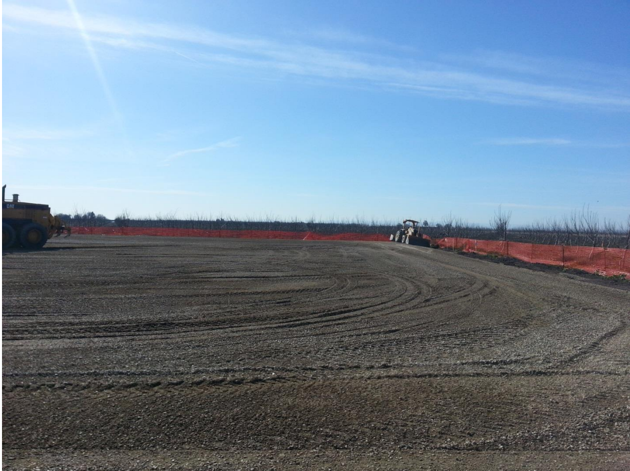
Figure 5-4. Aggregate Base Installed and Preliminary Compaction Achieved; Proof-rolling of Site Continues to Ensure Proper Compaction and Grading
