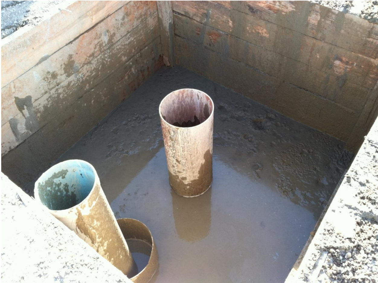
Figure 5-6. Conductor and Mousehole after Installation
