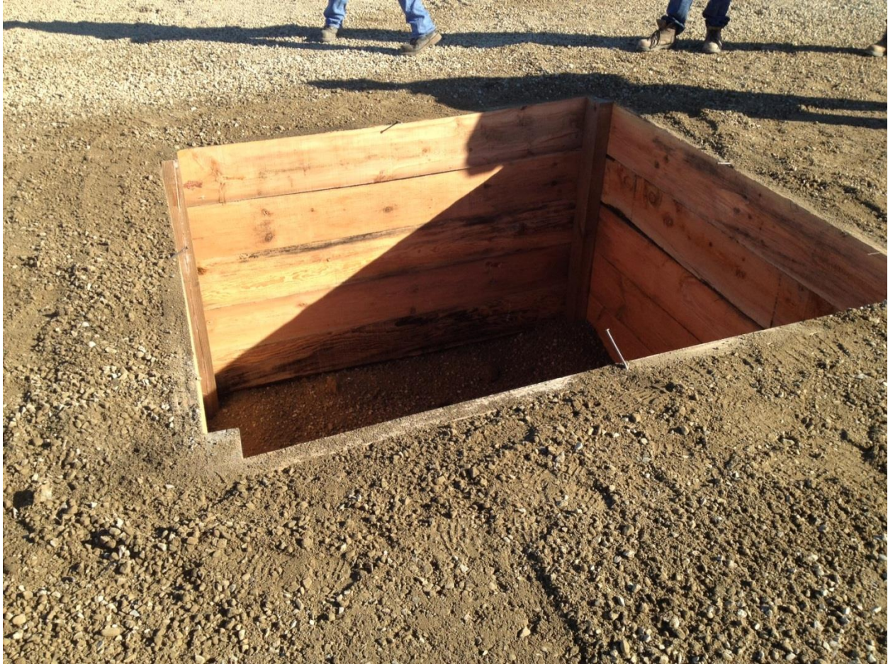
Figure 5-5. Cellar Installed (8 ft x 8 ft x 5 ft)
