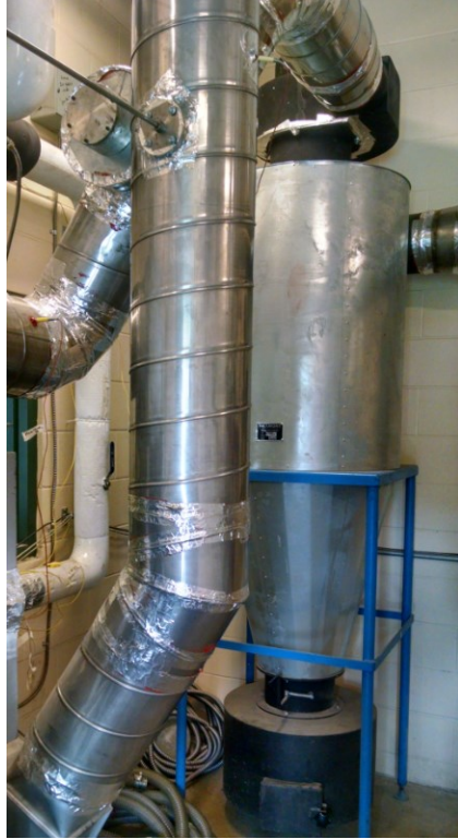
Figure 4 Cyclone dust collector installed at Clarkson University
