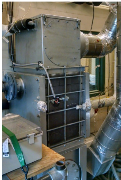
Figure 5 Condensing heat exchanger installed at Clarkson University
