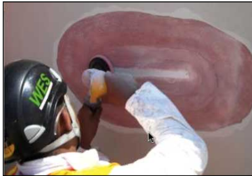
Scarfed Blade Repair Process
