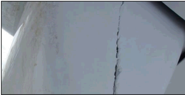
Severe Growth of Fiber Fracture
