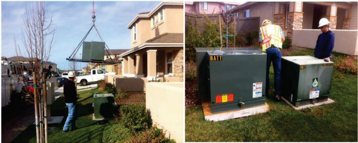
Figure 54. A 30-kW/34-kWh Distributed Energy Storage Unit (Being Installed and Inspected at the Sacramento Municipal Utility District's Anatolia SolarSmart Homes Development. Suppliers are SAFT, Grid Point, and Power Hub)
