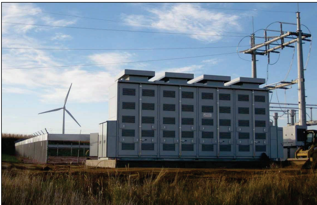
Figure 26. Xcel Battery Supplementing Wind Turbines, Lucerne, MN
