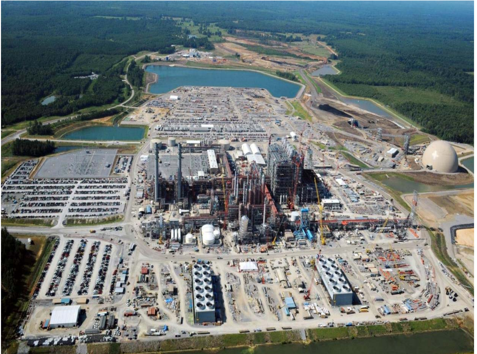
Picture F.3 - Overall site picture
