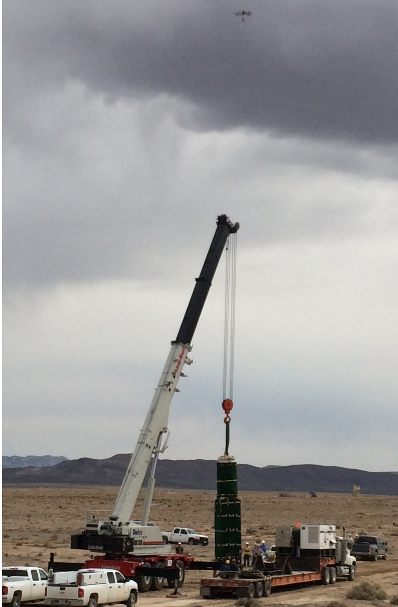
Figure 1: Photo of SH hoisted by crane
