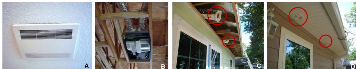
Figure 3-7. Ceiling-mounted energy recovery ventilator (A,B) installed in the main body with attic-mounted supply and exhaust ducts (B,C) terminating in soffit-mounted registers (D)
