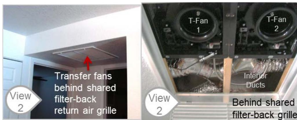
Figure 3-5. Southeast Volusia Habitat for Humanity home: transfer fans installed in the hall ceiling behind a shared filter-back return-air grille (left) in a small interior duct chase (right)
