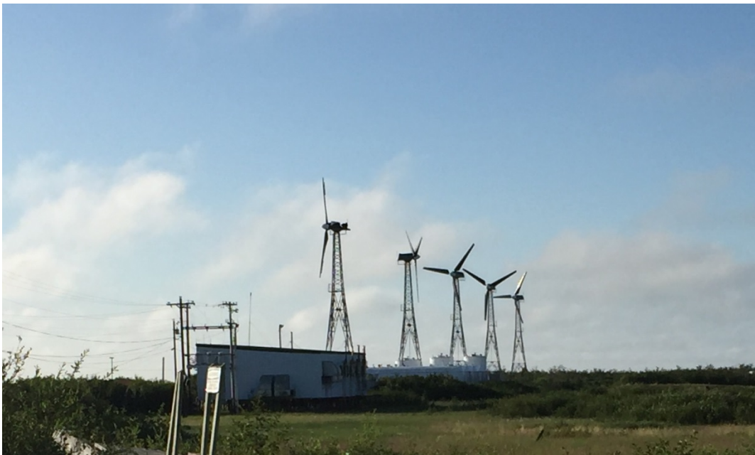
Tuntutuliak, AK - Five installed 95kW wind turbines as part of the Chaninik Wind Group
