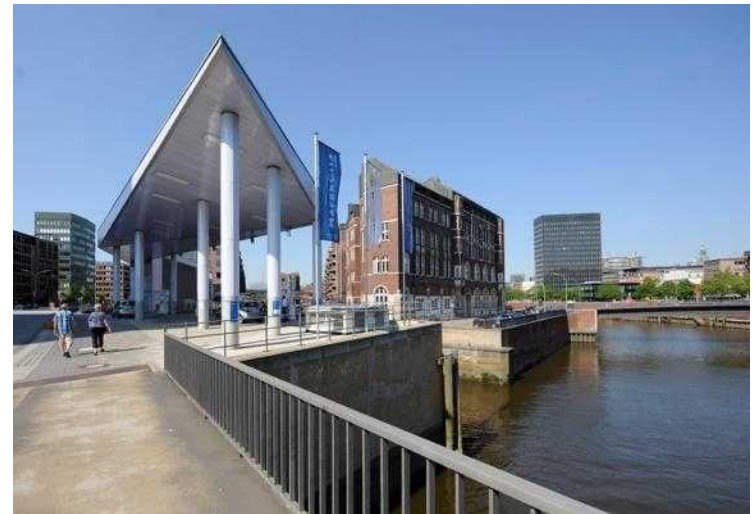
Example existing dockside hydrogen station in Hamburg, Germany
