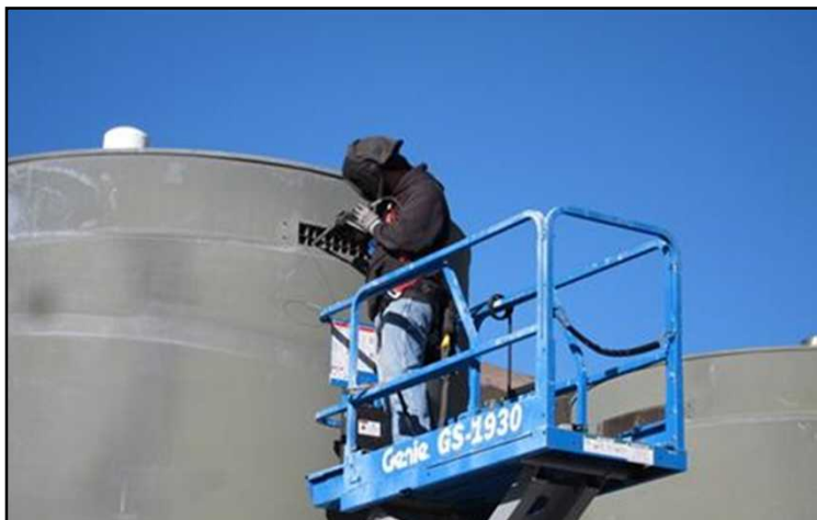
Removing the Gamma Shield
