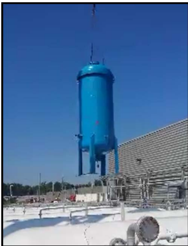
Figure 4. Spare carbon bed being lifted over CHL gas storage tanks for installation
