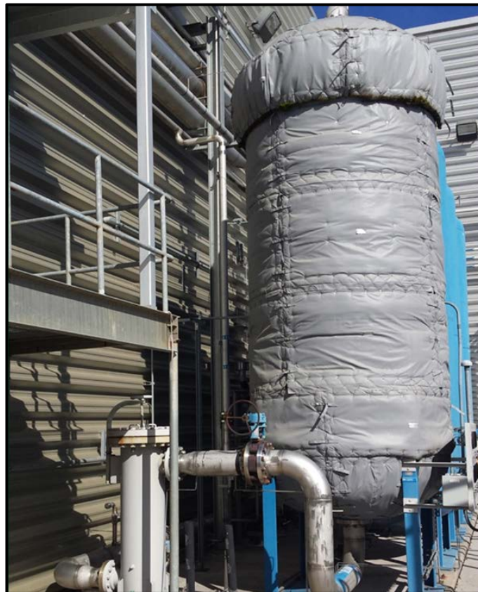
Figure 3. Existing CHL carbon bed vessel with heater blankets
