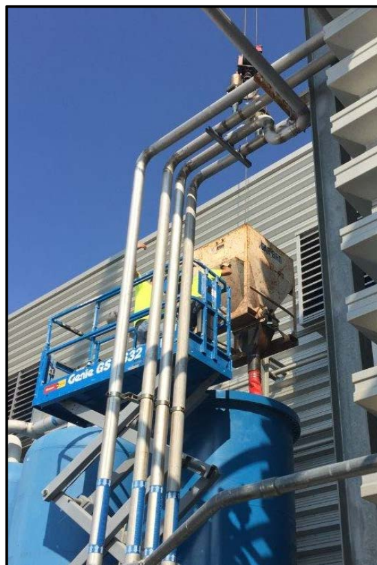
Figure 5. Crane lifted bucket for filling carbon media into vessel
