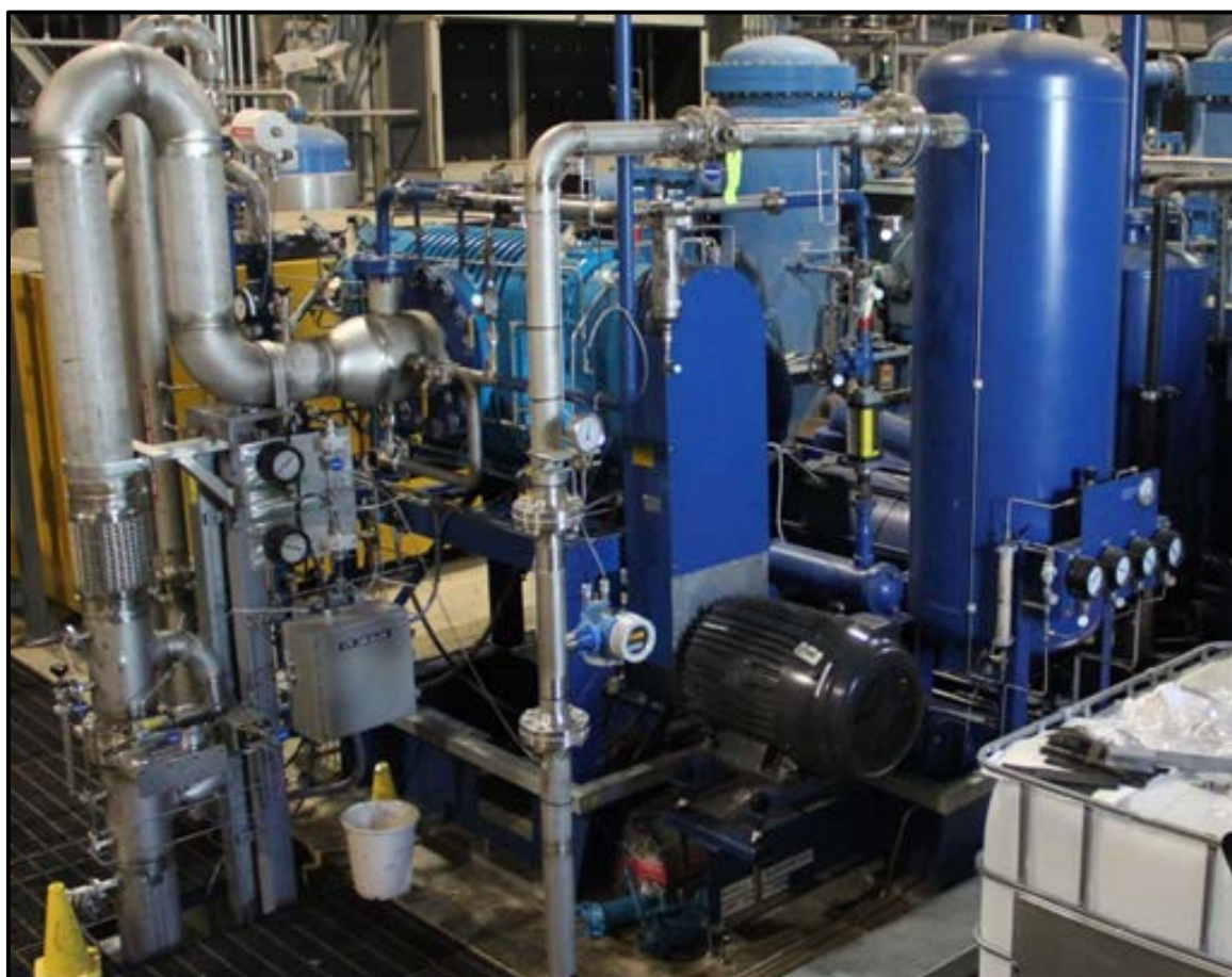
Figure 1. Operational Kinney pump skid connected to CTF piping
