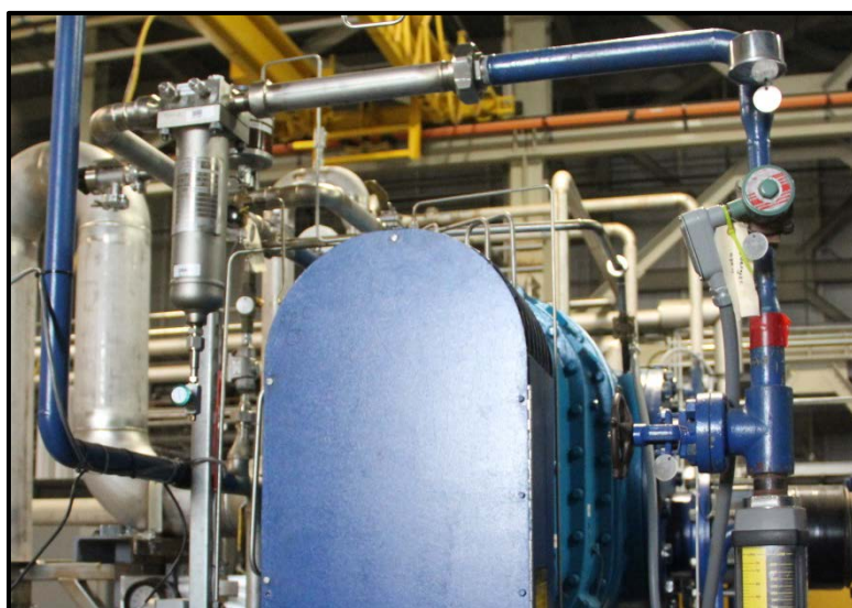
Figure 8. New filter element added to the Kinney blower oil injection line
