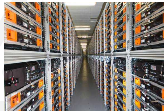
Tehachapi Wind Energy Storage Project - Southern California Edison Lithium-Ion Battery 8-MW / 4 hour duration
