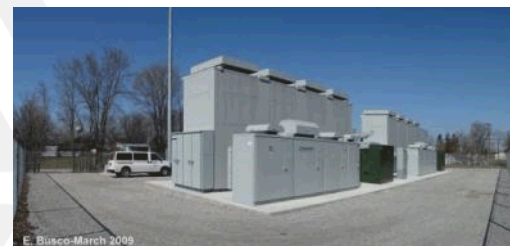
Sodium Sulfur Battery 2 MW / 8 hour
