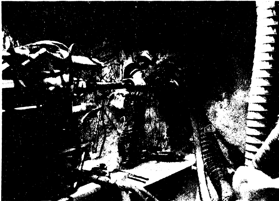
Figure 4.18-1. IS-2 overcore hole in Demonstration Drift (G-Tunnel) showing air-seal collar and dust suppression equipment.
