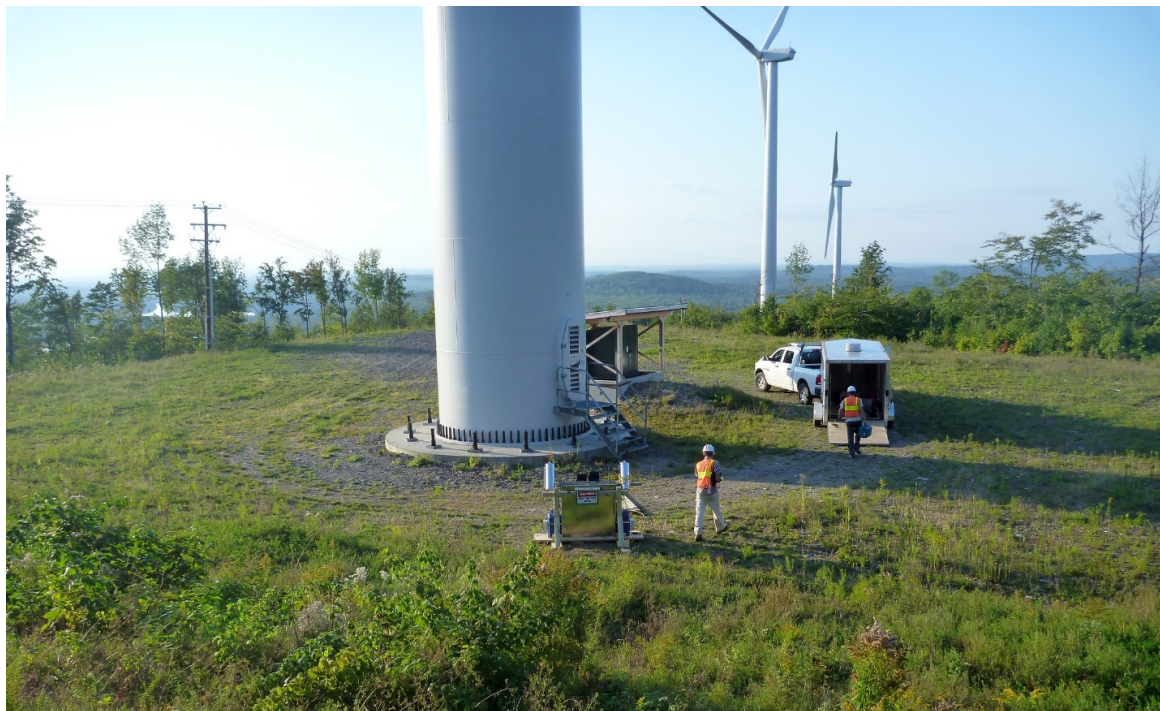
Figure 7. Camera installation at terrestrial wind farm.
