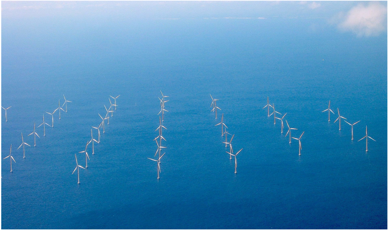
Figure 13: The Lillgrund Wind Plant
