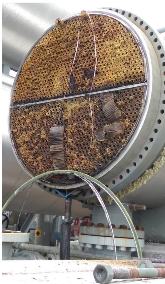
Figure 6. Dirty tube sheet for E-506 in December 2015
