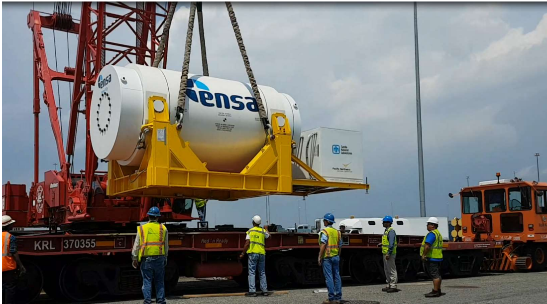
Image 7. KASGRO RAILCAR moved under cask immediately after SAMSON was removed from under cask. July/19 th
