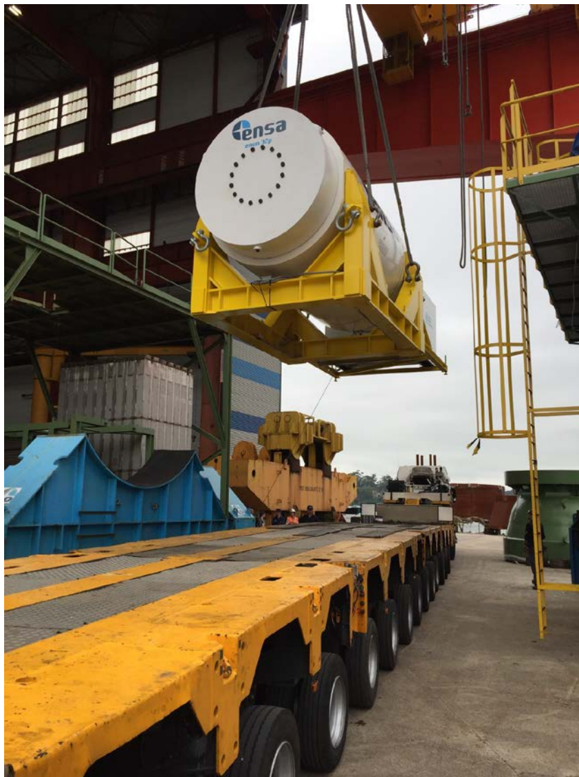
Figure 4-8. Lowering cask system on to Heavy-Haul Truck Trailer.
