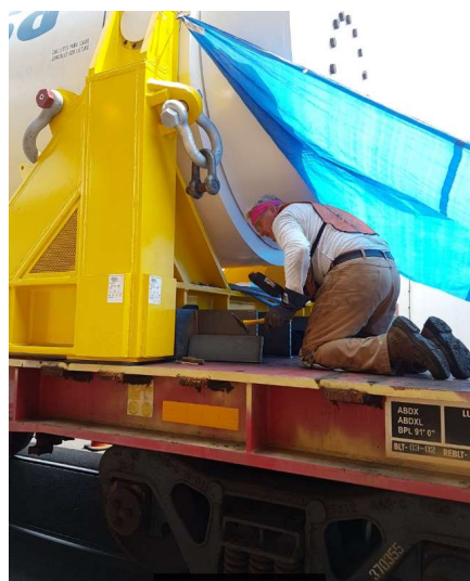
Image 11. Hot works start (welding stoppers). July/20 th
