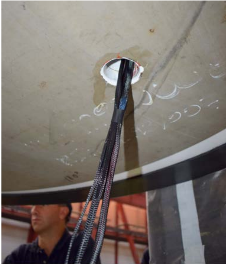
Figure 3-8. Placing instrumentation cables through lid.
