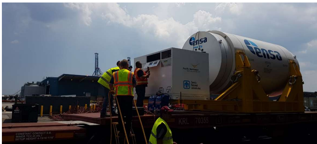
Image 10. SANDIA/PNNL staff connecting chargers to the batteries. July/19 th
