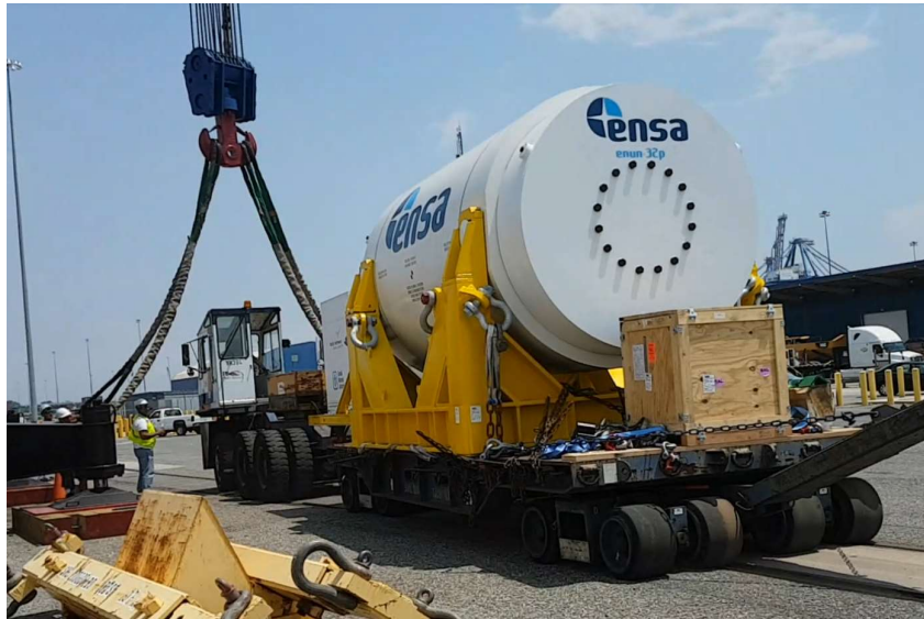
Image 3. Tug master and cask on SAMSON being moved under crane's hook. July/19 th
