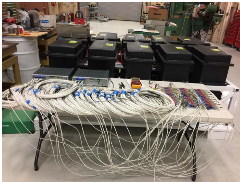
Figure 3-26. Siemens LMS SCADAC 5-slot Recorders with LMS SCADAC Mobile 8-channel universal durability input modules, instrumentation cables, junction panels, and batteries used to power the data acquisition system.
