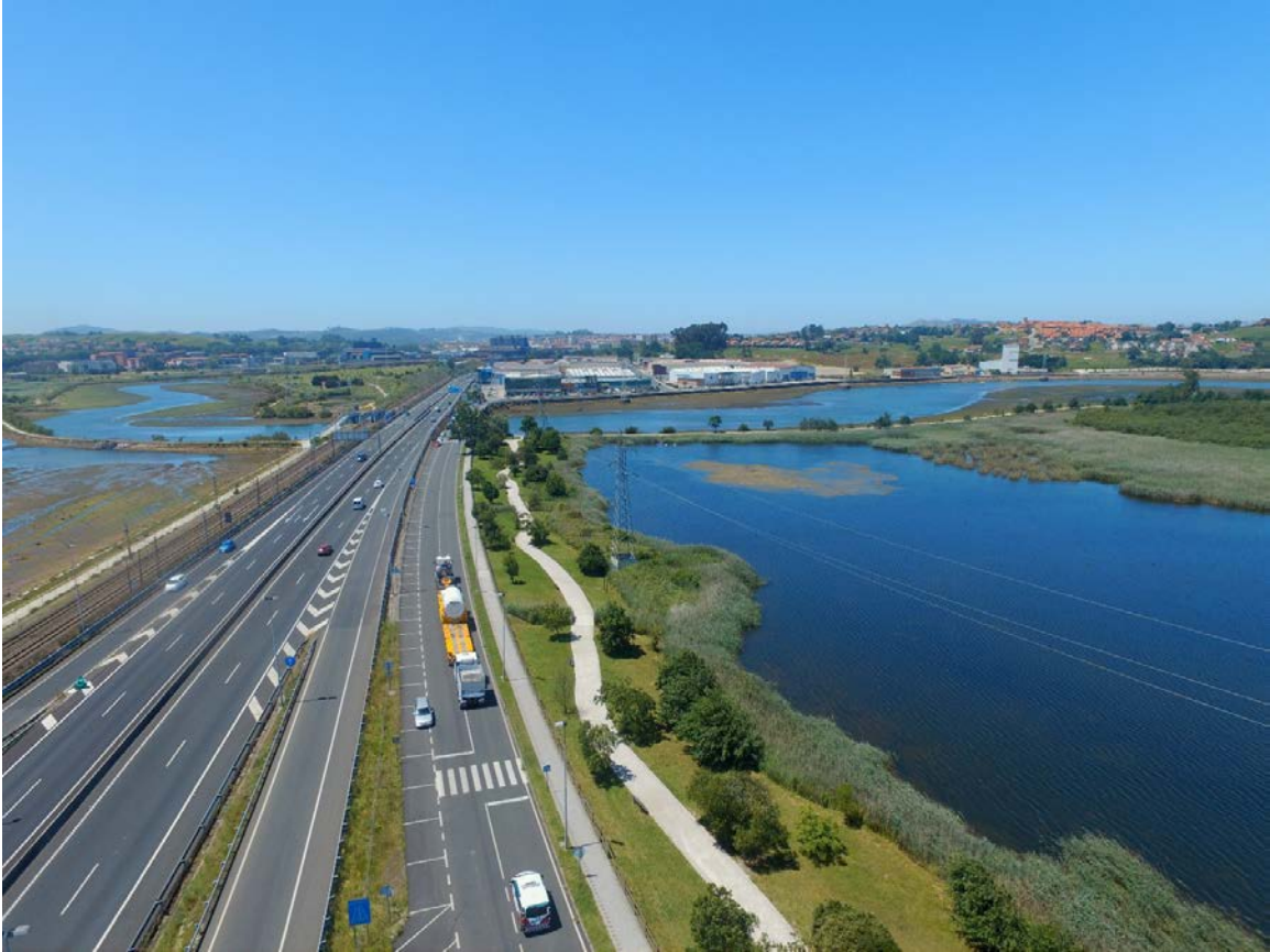
Figure 4-17. Heavy-haul truck transport.
