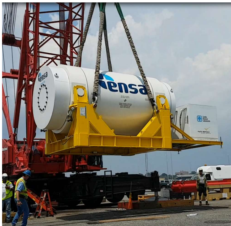
Image 6. SAMSON removed under CASK and CASK lifted waiting for railcar to be moved under it. July/19 th
