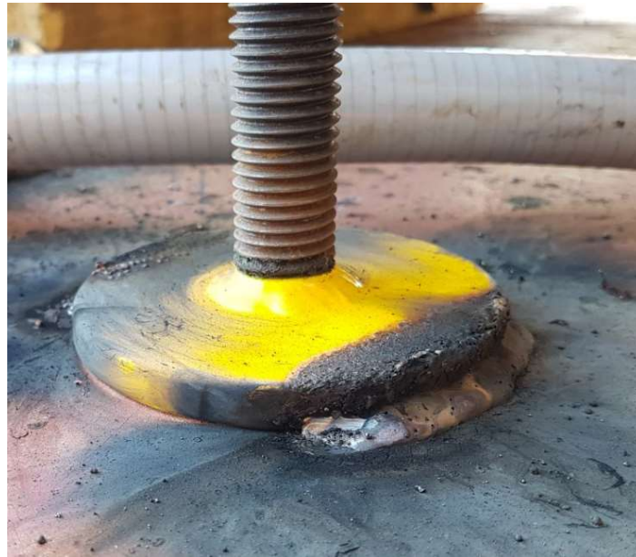
Image 19. Leg for supporting cradle for batteries was welded to avoid background vibrations.
