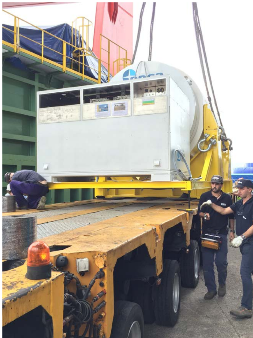
Figure 4-9. Lowering cask system on to Heavy-Haul Truck Trailer.
