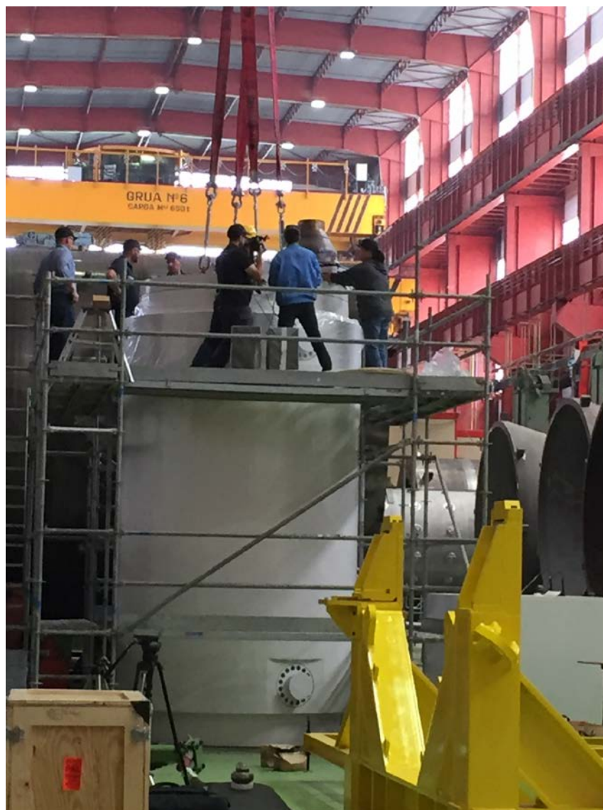
Figure 3-33. Placing the instrumentation lid on the cask.
