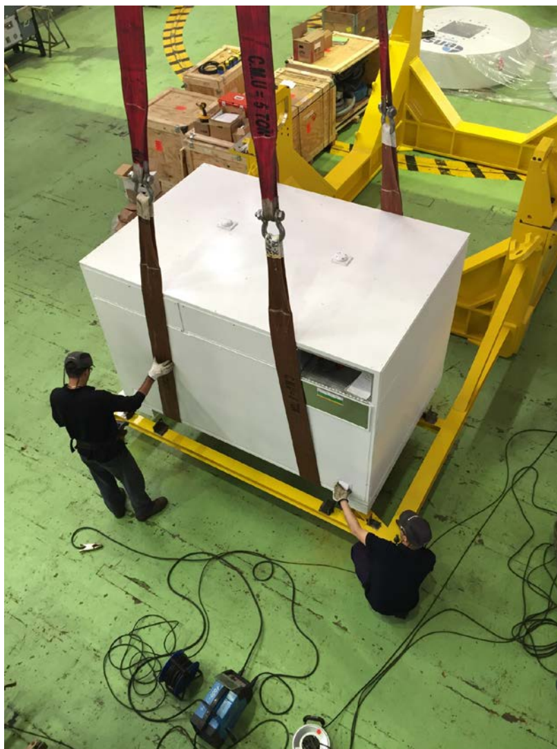
Figure 3-36. Data Acquisition/Battery Box being placed onto cradle.
