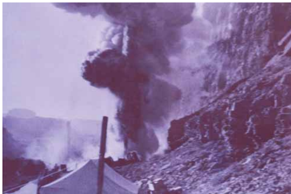
Figure 14. Drilling on the axis of the Cane Creek anticline along the banks of the Colorado River in the 1920s. Material was floated down the river on barges and the rig and houses were constructed on site. The well blew out while drilling in the upper Paradox Formation. Photographs from the Utah Historical Society.
