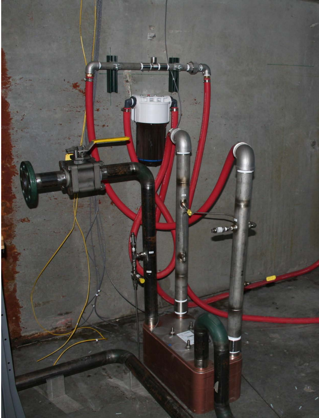
Figure A6. Heat exchanger (bottom of photo) along with piping and instruments. A water filter is mounted on the wall near the top.
