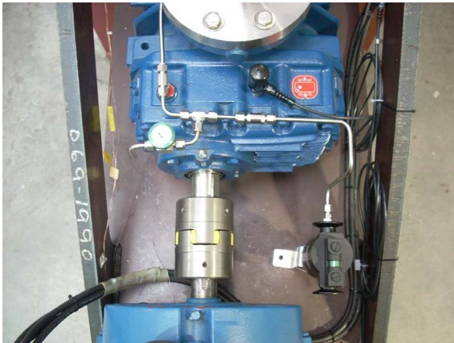
Figure 16 – Installed pressure relief system to relieve pressure from the blower gear boxes.
