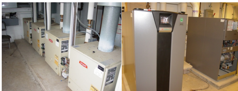
Figure 7: Typical boiler installations in buildings at Camp Dawson.
