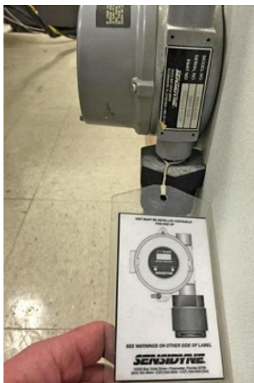
Figure 2.3.1-3 - Details of the CO 2 sensor used.
