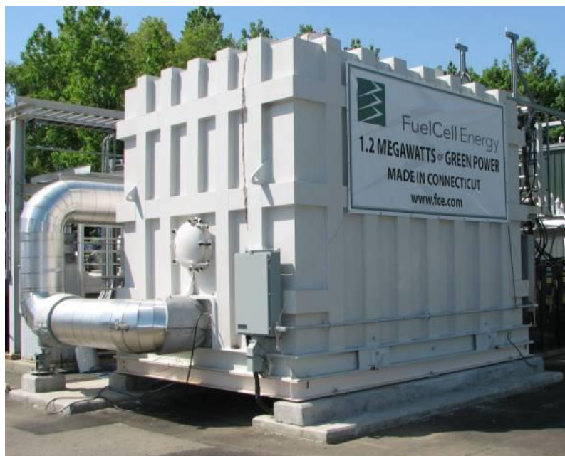
Figure 1-2. Typical MW-scale Fuel Cell Module (a major component of the FCE power plant product called DFC1500)
