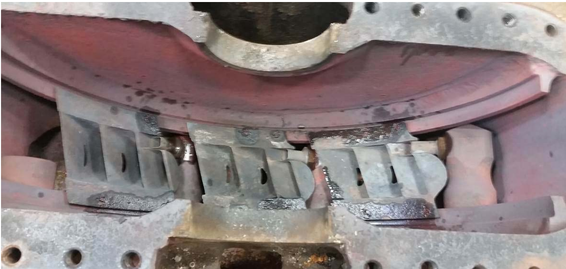
Figure 39 Lower casing, with original nozzles and reversing chambers
