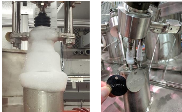
Figure 7. Ice formation on the cryomodule JT valve and Distribution Box Instrument Line
