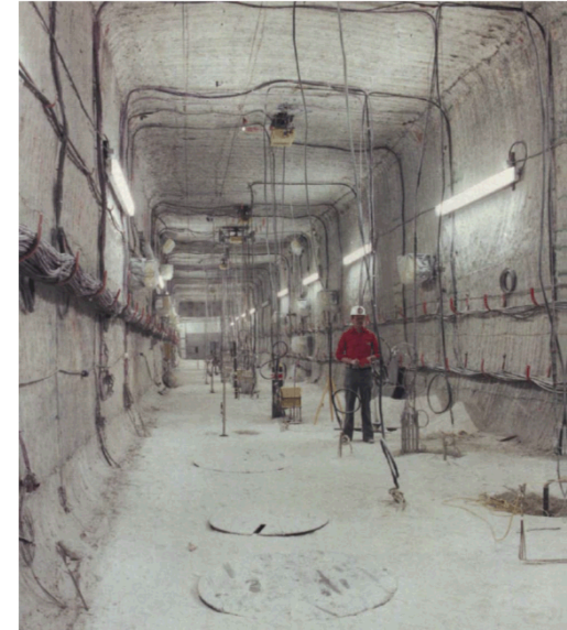
Heater Tests in WIPP Room B, 1985 from Matalucci 1987, SAND87-2382
