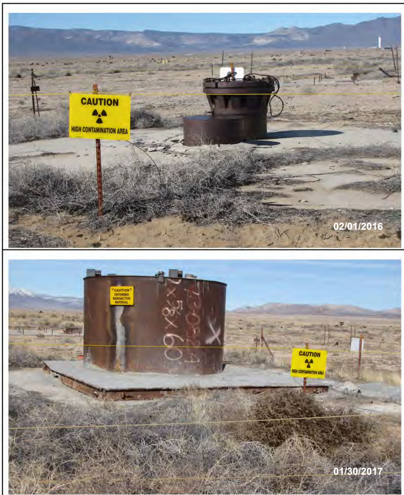
Figure 2-4 San Juan Well Head Assembly before and after Corrective Action
