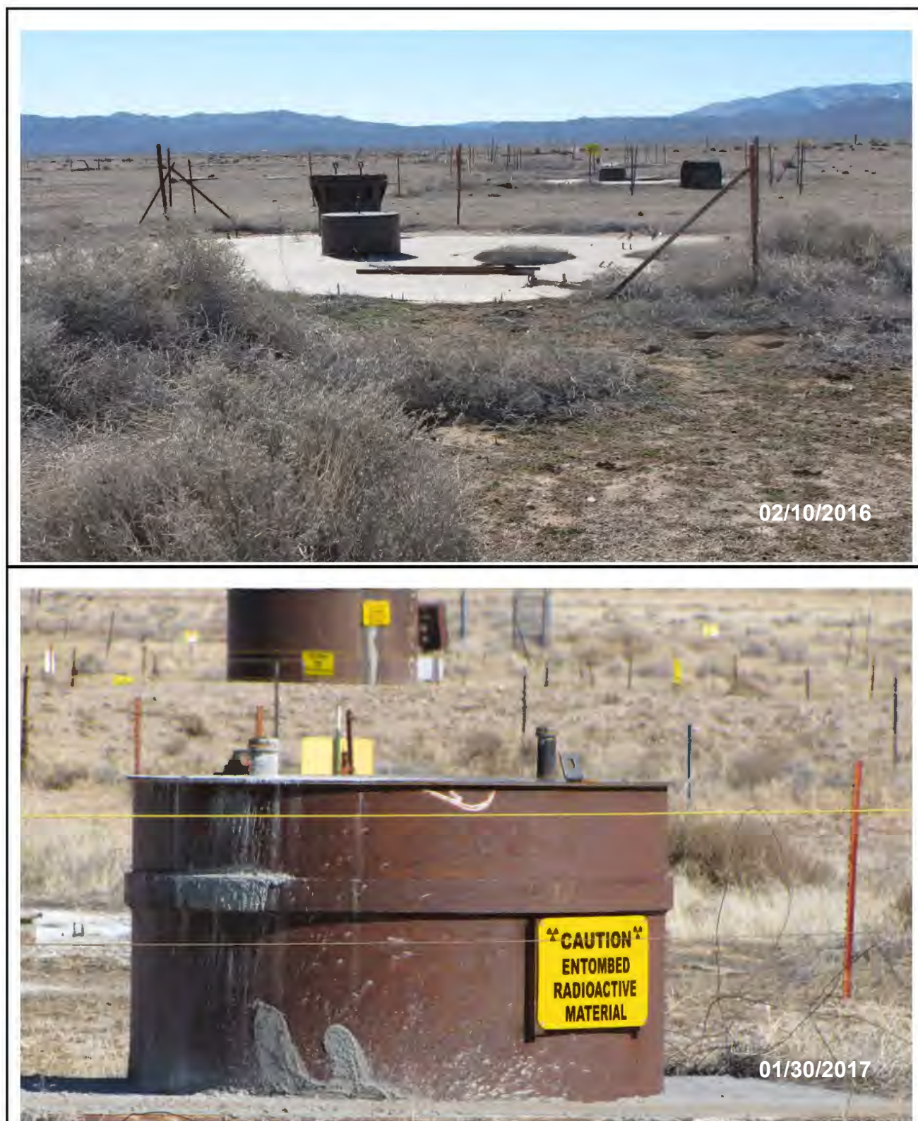
Figure 2-7 Luna Well Head Assembly before and after Corrective Action
