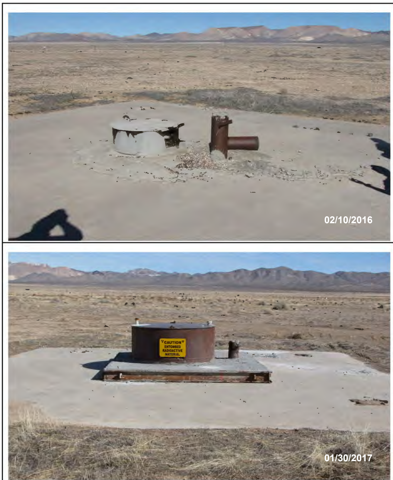
Figure 2-9 Pascal-A Well Head Assembly before and after Corrective Action
