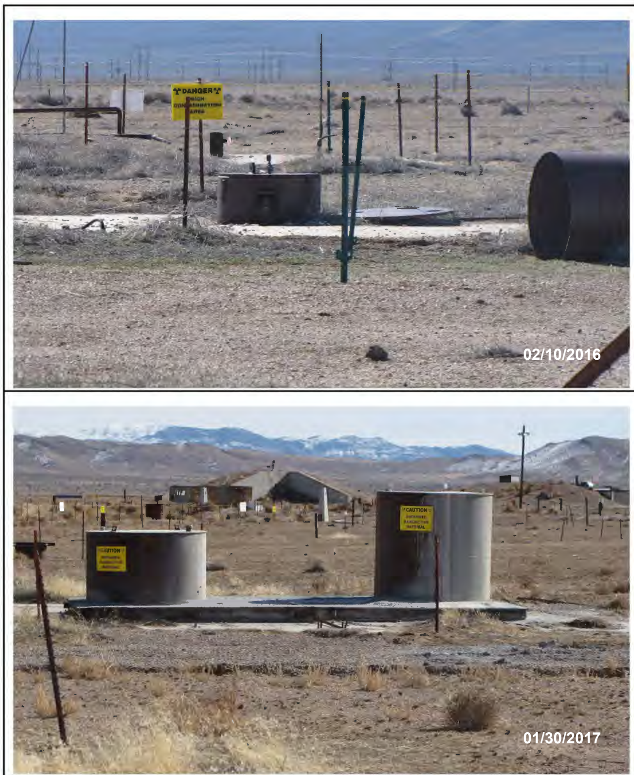
Figure 2-6 Pascal-B Well Head Assembly before and after Corrective Action
