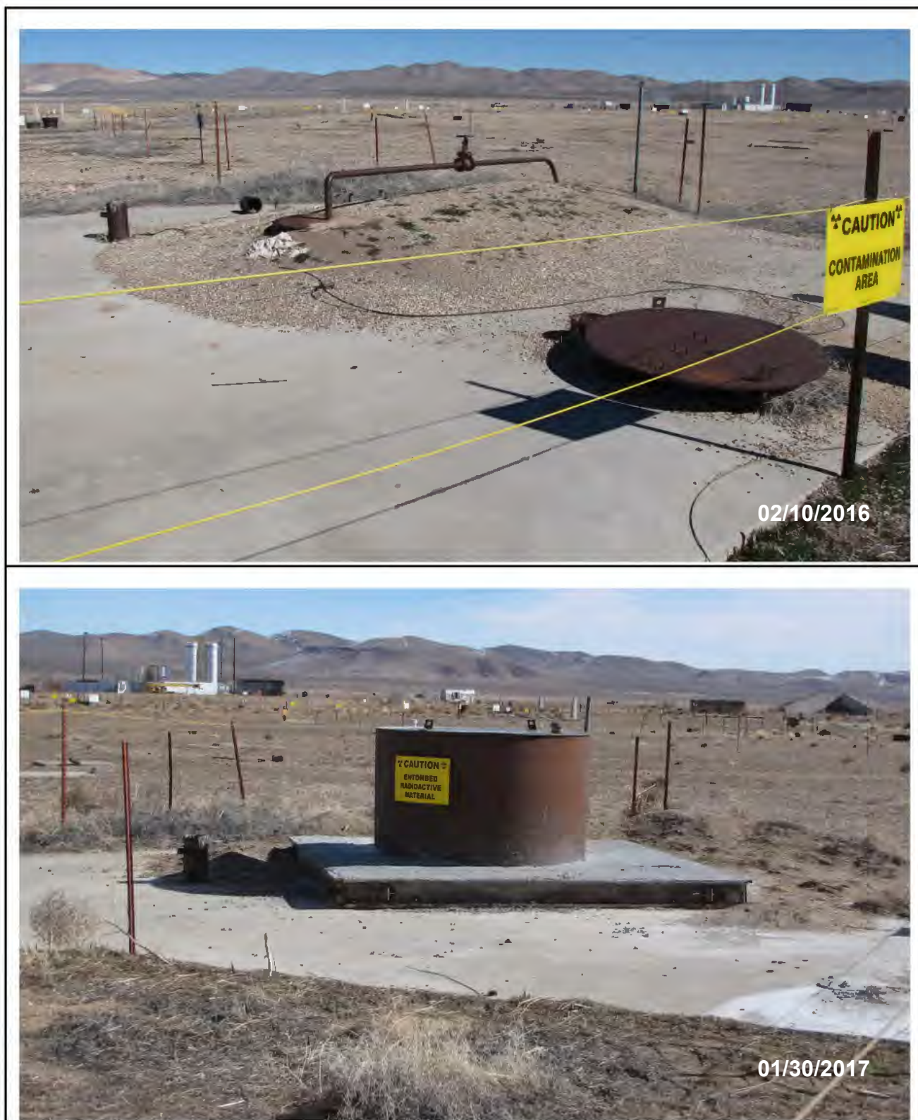
Figure 2-8 Colfax Well Head Assembly before and after Corrective Action
