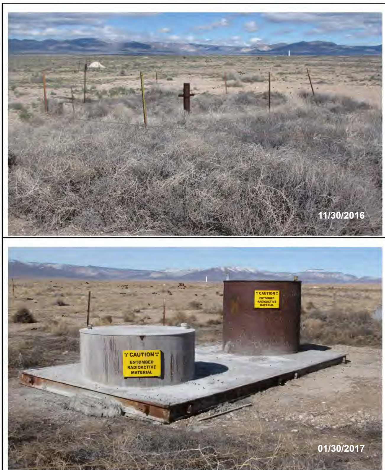
Figure 2-5 Pascal-C Well Head Assembly before and after Corrective Action
