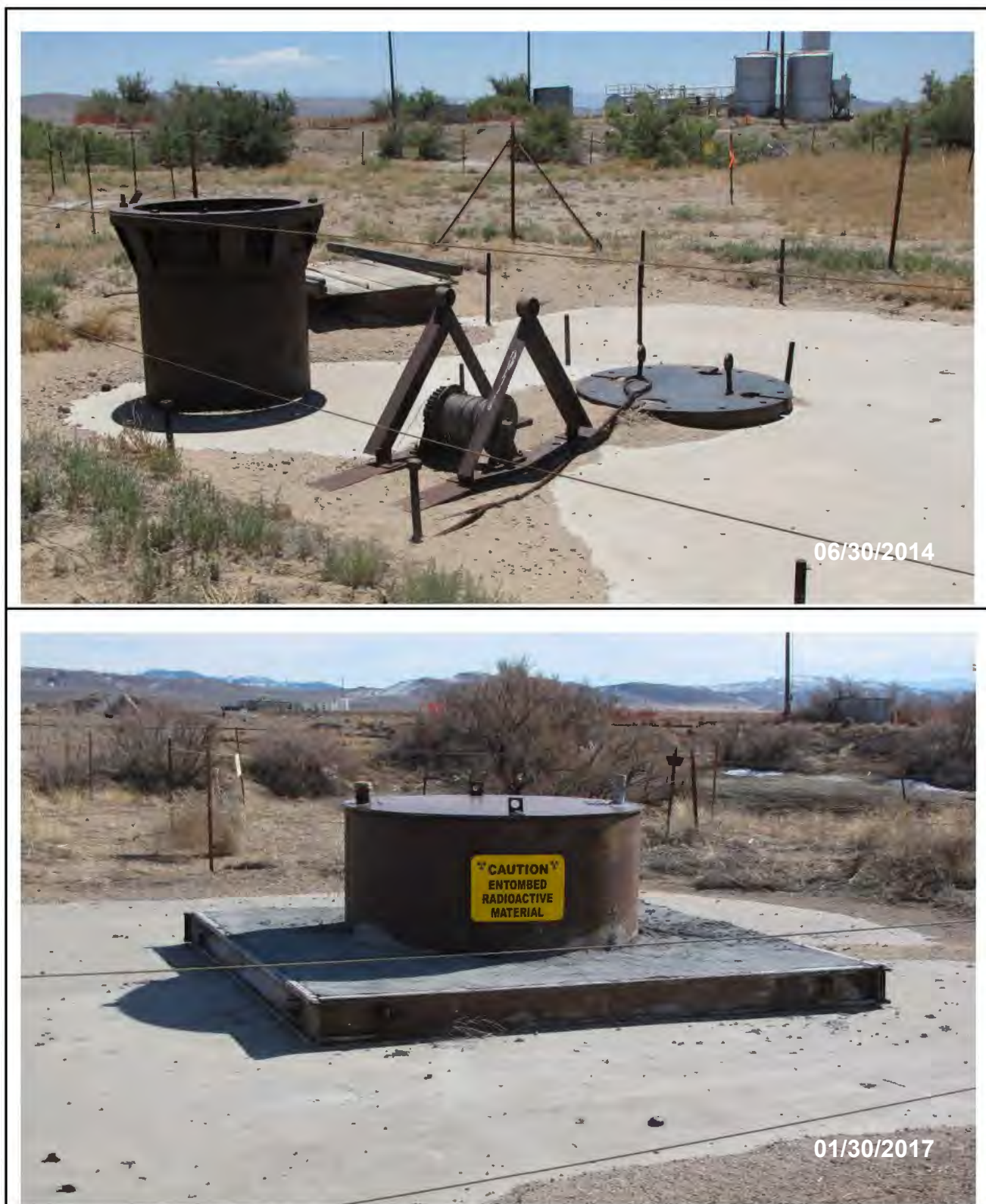
Figure 2-10 Valencia Well Head Assembly before and after Corrective Action
