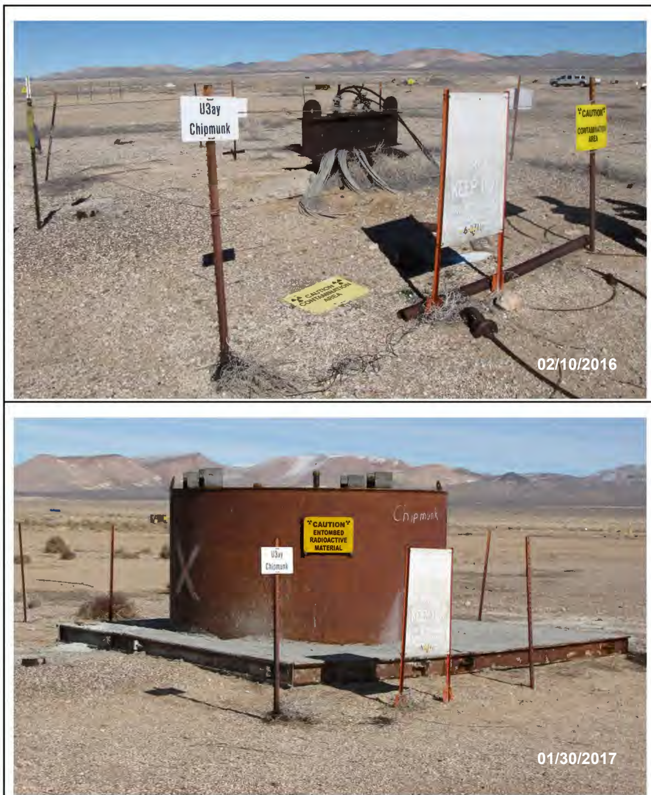
Figure 2-11 Chipmunk Well Head Assembly before and after Corrective Action
