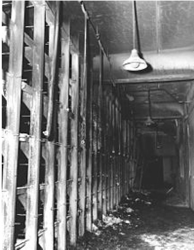
Figure 2 Rocky Flats radiological filter bank after catastrophic fire (Source: Department of Energy)
