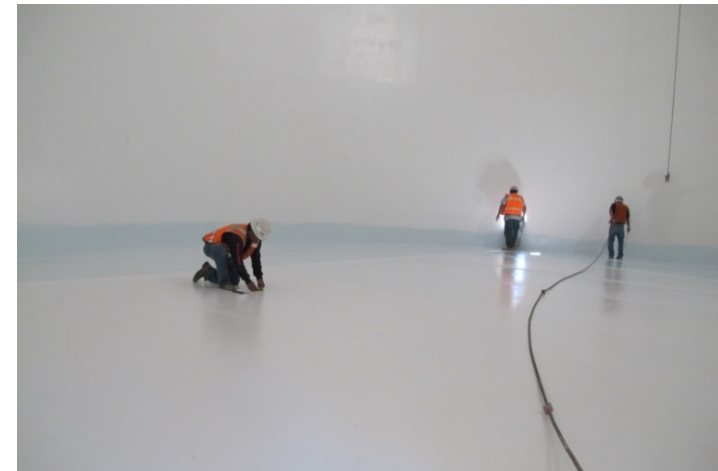
Water tank interior after renovation
