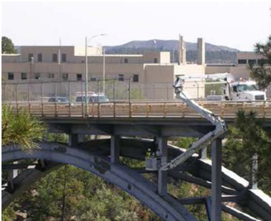
Annual bridge inspection evaluation of superstructure
