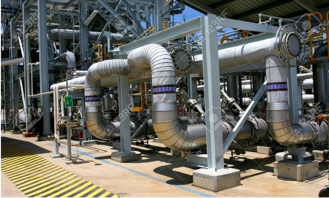
Figure 15. Example of a manifold for steam distribution.
