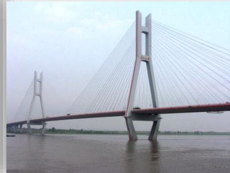
The Wuhan Junshan Bridge over the Yangtze River is covered with 35,000 m 2 (~8.5 acres) of thermal sprayed zinc coating!
