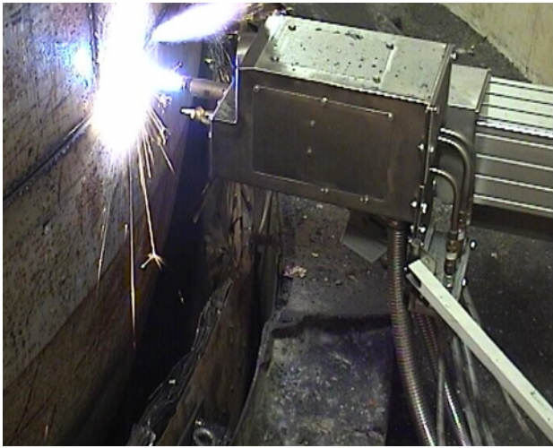
Fig. 4. Vertical cut using an oxy-propane torch of a Zion Unit 1 RPV Level 2 Segment [15].
