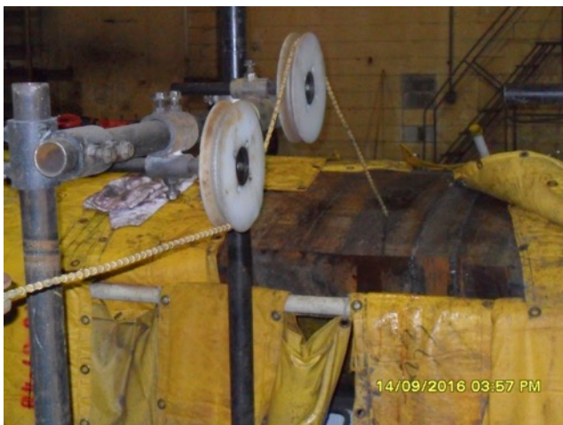
Fig. 13. Wire saw cutting parallel to the beltline weld [15].
