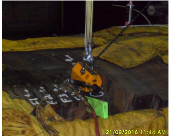
Fig. 14. Lift magnet used to remove the cut blocks [15].
