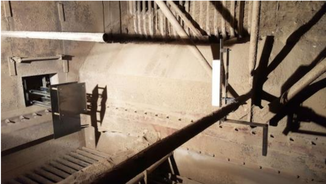
Figure 55: Modified interrogating antenna and a new sensor package installed in the economizer.
