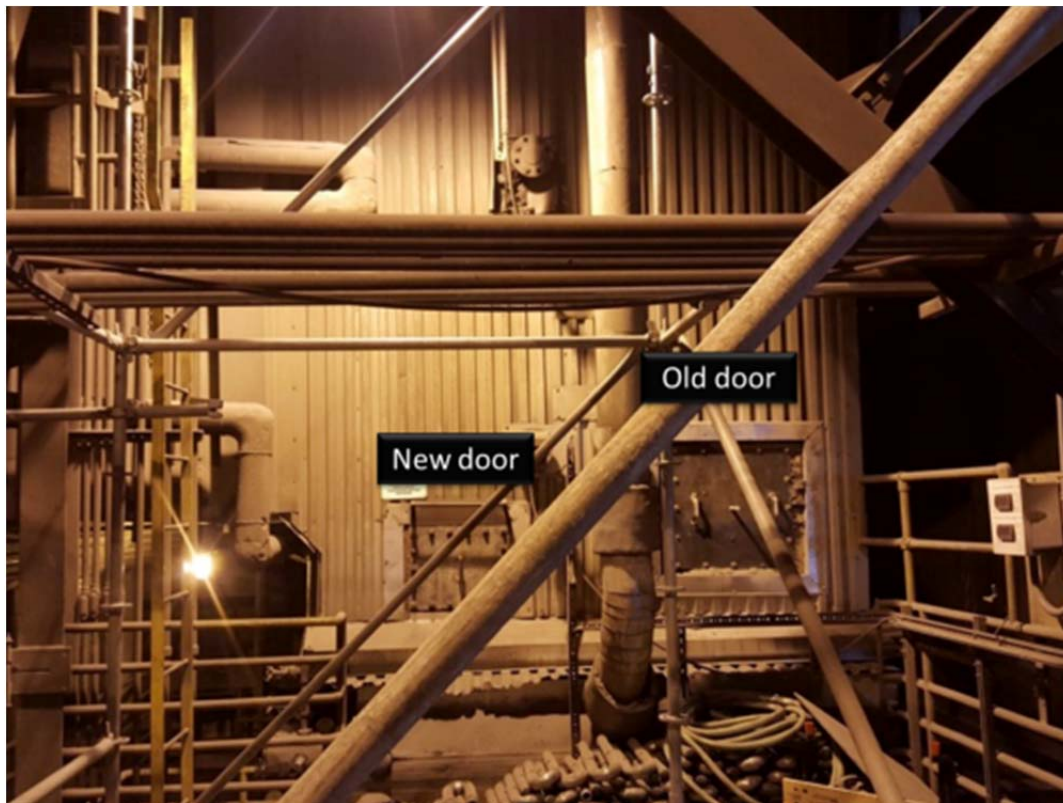
Figure 49: The new door location indicated in the picture served the purpose of housing the interrogating antenna for the boiler sensor array.
