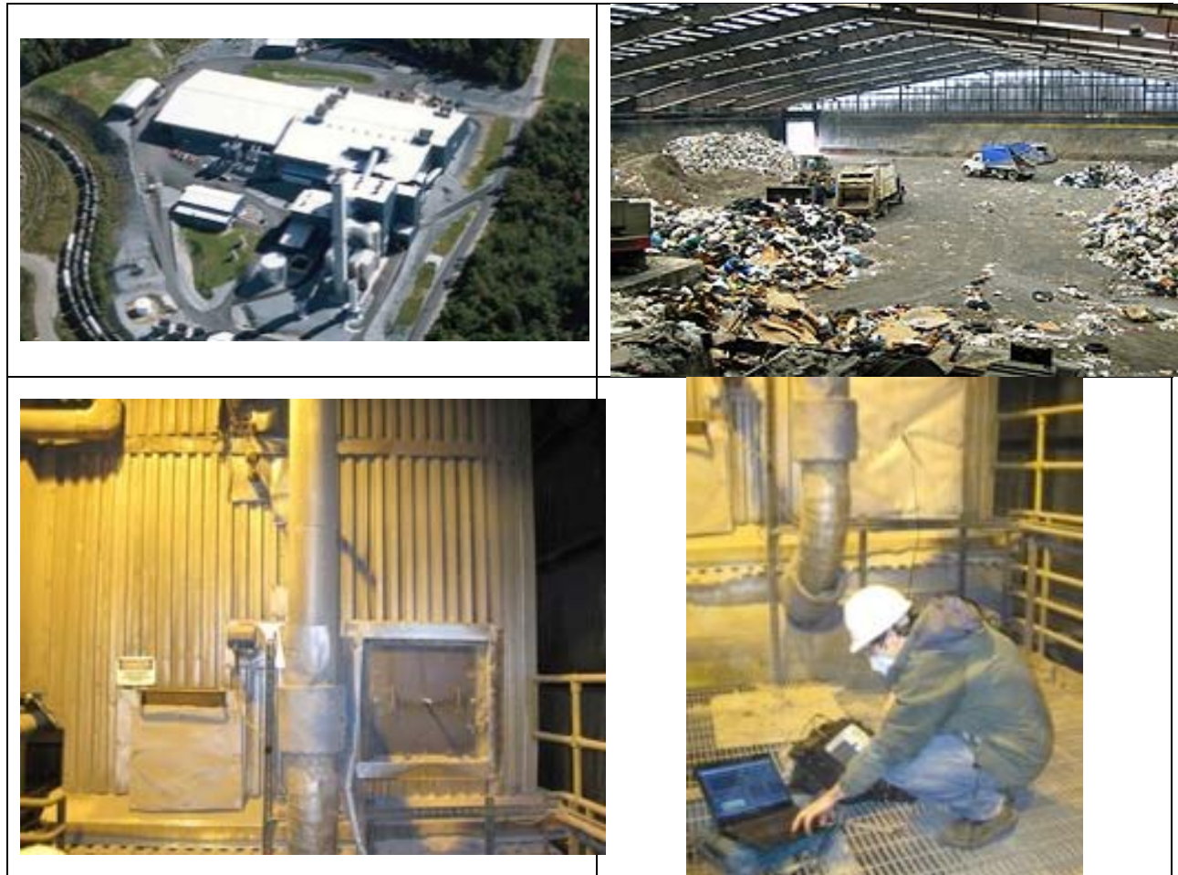
Figure 11: (Top-left) Penobscot Energy Recovery Company (PERC) power plant facility; (Top-right) Garbage separation in preparation for burning; (Bottom-left) Back of the boiler section and economizer region, with access port, where different wireless sensor array architectures were tested; (Bottom-right) Environetix engineer performing a wireless SAW sensor array routine monitoring.
