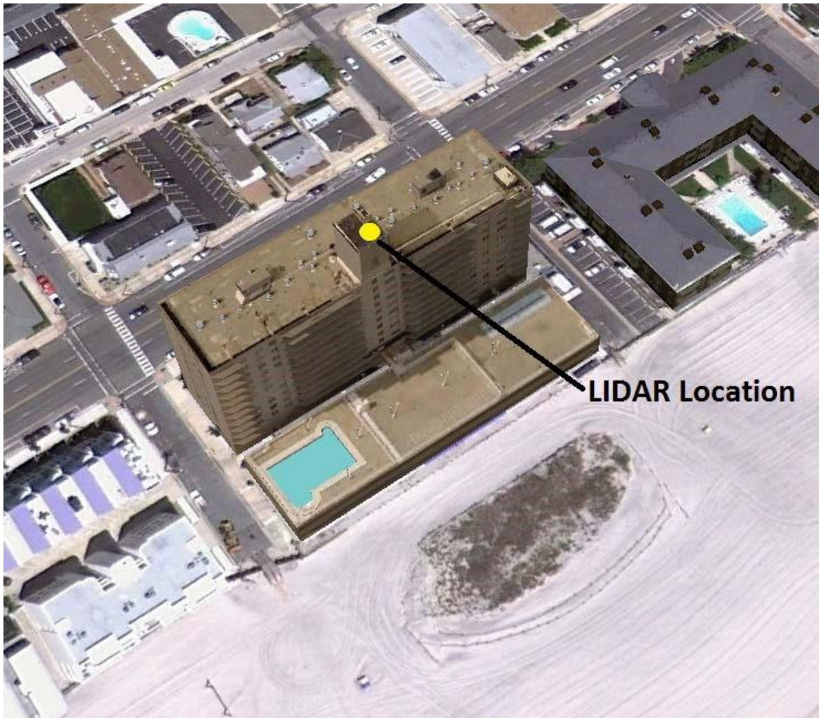
Figure 2. Location of WindTracer LIDAR on top of the elevator shaft of the Margate Towers Condominium Building in Margate, NJ.
