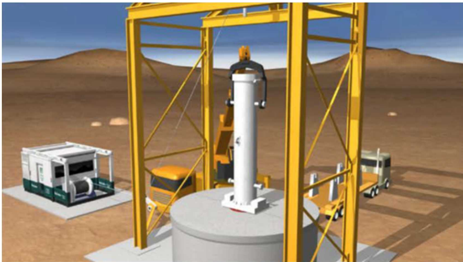
Crane placing loaded transfer cask on wellhead (SNL 2016).
