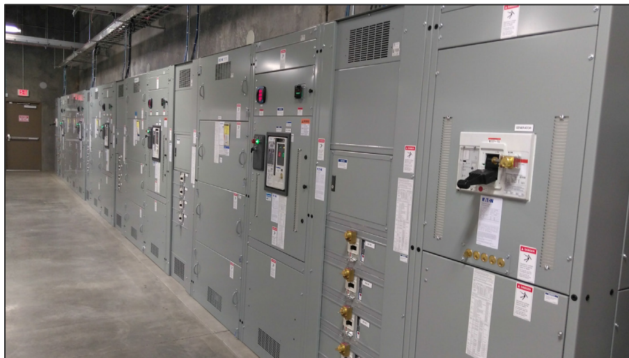
Figure 3.6. BESS Panels
