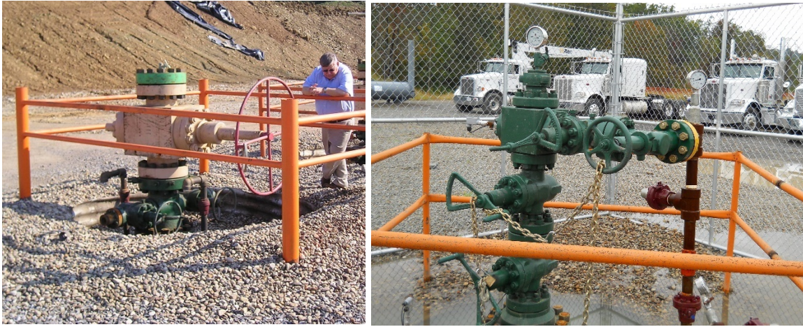
24. Photographs of a massive fracture gate wellhead on a recently drilled Marcellus Shale well in Greene County, Pennsylvania, prior to hydraulic fracturing (L), and a production wellhead (i.e., Christmas tree) on a producing Marcellus Shale well (R). Photographed by Dan Soeder in 2011.
