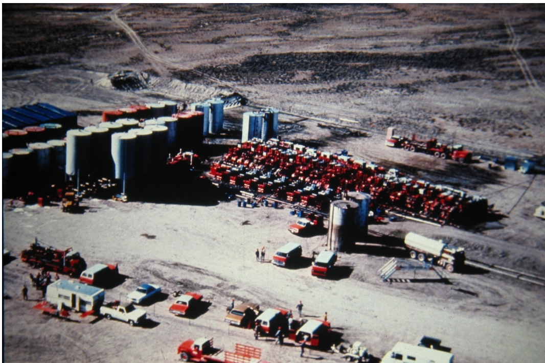
14. Photograph of the massive hydraulic fracture operation on the El Paso Natural Gas Wagon Wheel well near Pinedale, Wyoming in 1974; photo courtesy of Phil Randolph.
