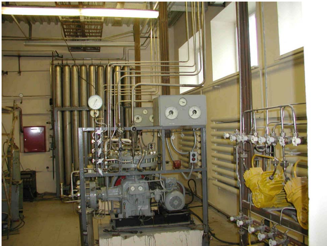
Picture 2: Pumps for circulating the Liquid Nitrogen coolant for the distillation of CO.
