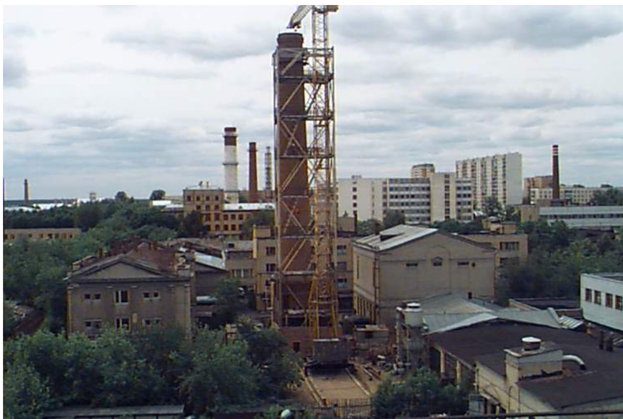
Picture 1: View of the cryogenic distillation tower at the Kurchotov Institute for isotopic separation of the carbon isotopes through the cryogenic distillation of CO.
