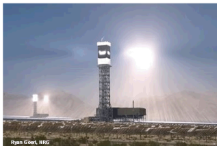
FIGURE 1. Left: Illumination of standby heliostat aim points next to the receiver at Ivanpah. Right: Grid of prescribed bird flight paths in the irradiated region that are used to assess potential avian flux hazards in this study.
