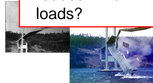
Tacoma Narrows Bridge collapsing under 40 mph winds (1940)
