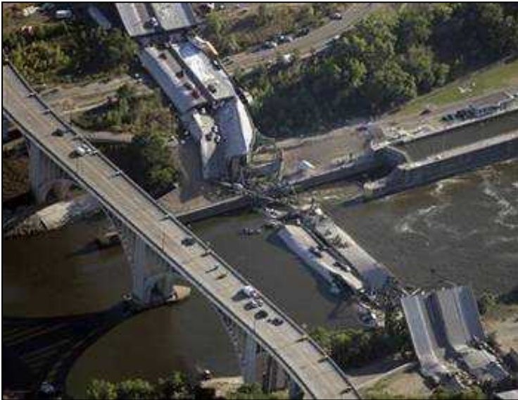
Monitor Bridges – Interstate 35 Failure in USA
