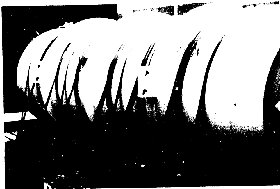
Figure 7. Steel strap tie-downs
