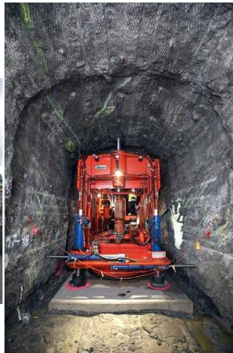
Boring of deposition holes
