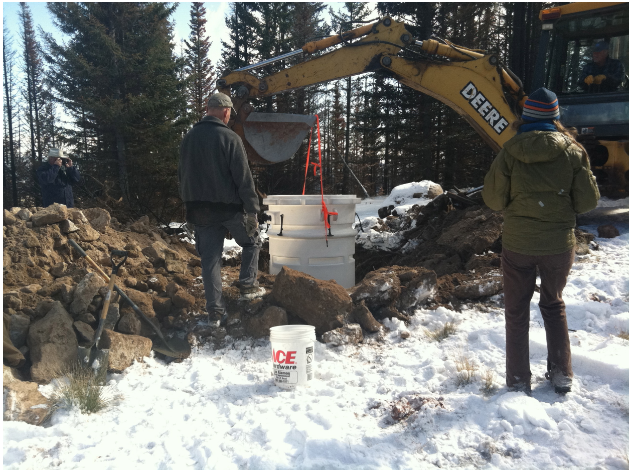
Figure 4: Plastic vault barrel being installed in excavated hole at station CDAB.
